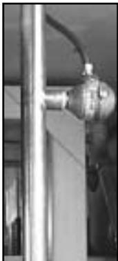
Pictured at the left is a SFI installed in a plant that manufactures ink for desktop printers and copy machines. 100-pound batches of carbon black come out of a feeder and are pneumatically conveyed through a four-inch vertical line. The SFI is used to indicate when a batch of carbon black has cleared the line.
